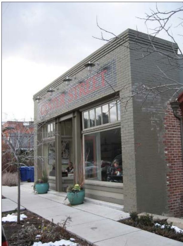
This one story building at 271 N. Center Street (c. 1900) is an example of a one-part commercial block.
