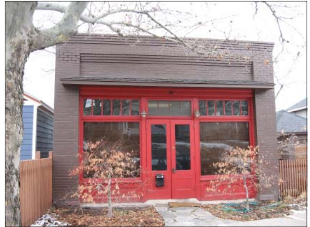
Woodwork is a character-defining feature of this storefront at 361 N. Main Street.
