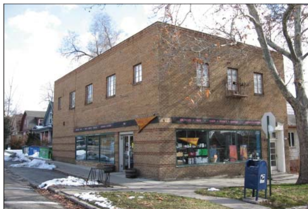
The building at 702 E 3rd Avenue (ca. 1940) was designed with simple detailing and has rectangular steel casement windows and original display windows.
