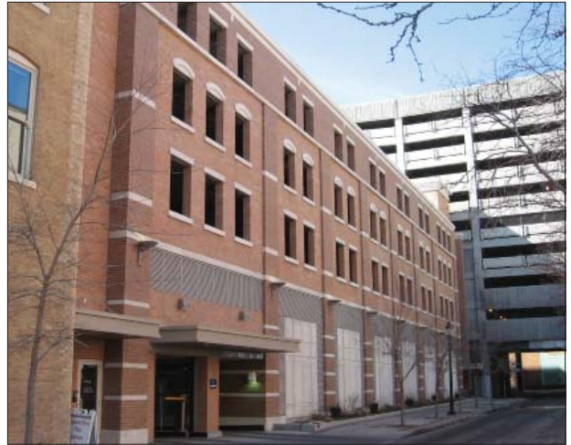
Site multi-story parking lots in the downtown area at interior areas of the block; design them to screen vehicles as much as possible, such as this garage in the 100 block of State Street.
