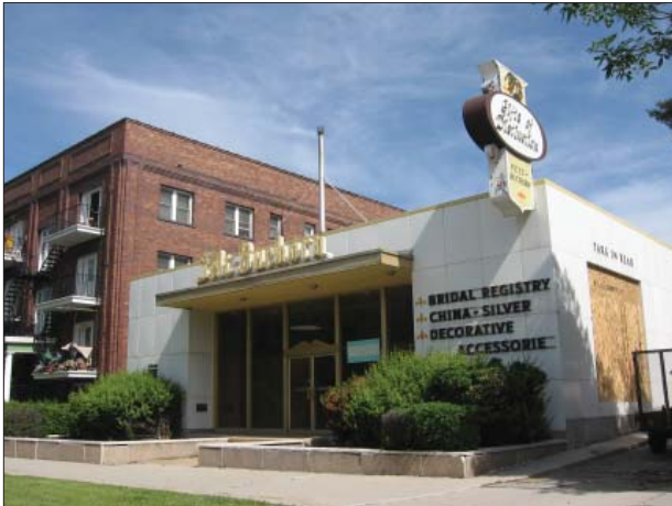
An enframed window wall plan is the Felt-Buchhorn Building at 445 E. South Temple Street (1959). It displays a continuous surround of porcelain steel panels which frame the display windows and entrance.
