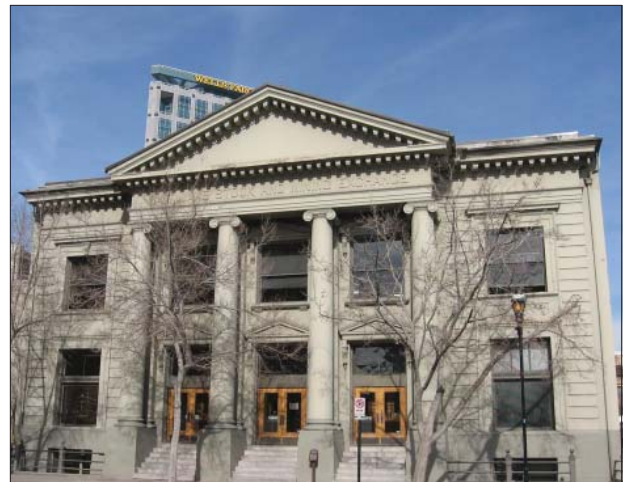
The Salt Lake Stock and Mining Exchange at 39 Exchange Place demonstrates the Neoclassical style with prominent classical columns and accentuated entrances.
