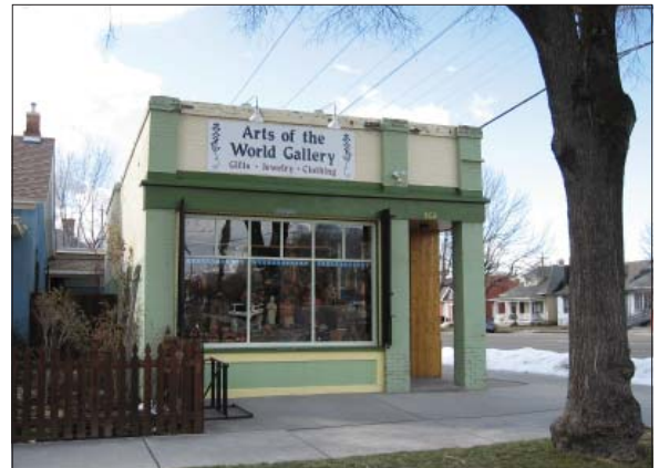
A simple one-part commercial block at 779 South 500 East.
