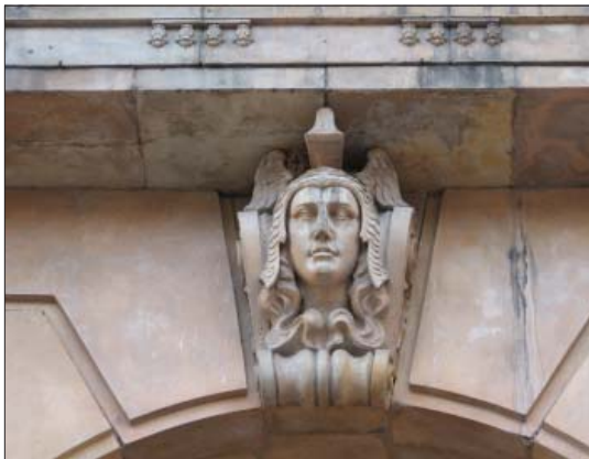
Decorative keystone of the Commercial Club Building at 32 Exchange Place.
