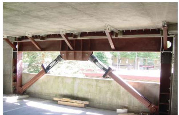
Seismic retrofitting can include adding steel frames and dampers in basement and parking areas of commercial buildings.
