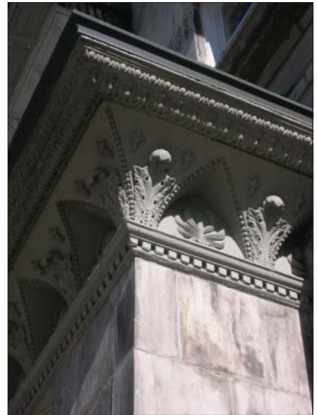
Decorative embellishment plays a significant role in the facade composition of the Alta Club at 100 E. South Temple Street.
