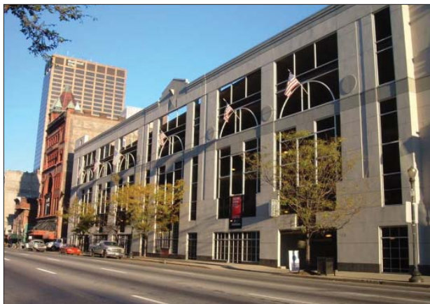
When built directly on the street, design new parking garages to complement adjacent historic buildings in materials, fenestration and overall design.
