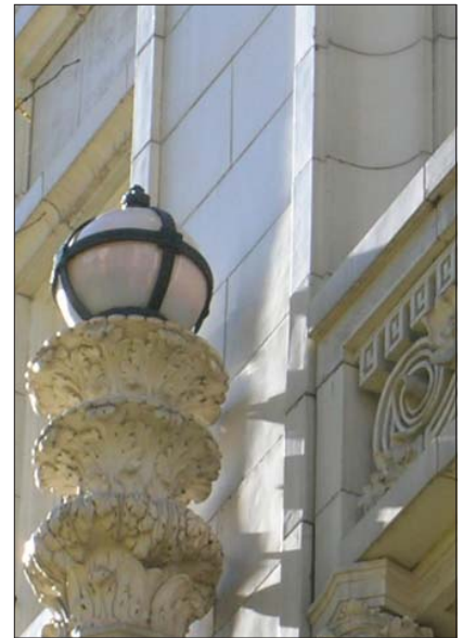
Historic lighting provides distinctive detail to the Kearns Building at 136 S. Main Street.
