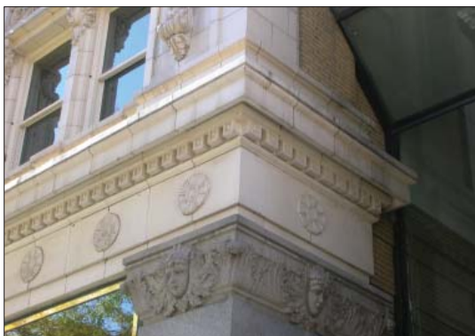
Molded terra-cotta rosettes adorn the facade of the Kearns Building at 136 S. Main Street.
