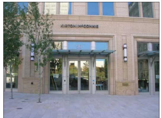
Canopies provide shelter of the public, can be used to define an entry and add interest to a building facade.
