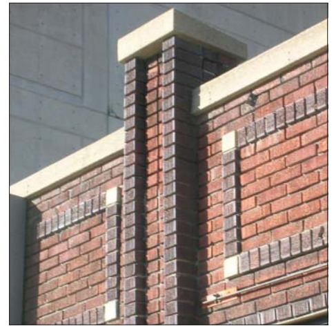
Variations in brickwork color, texture and pattern can provide interest to a relatively simple street facade.
