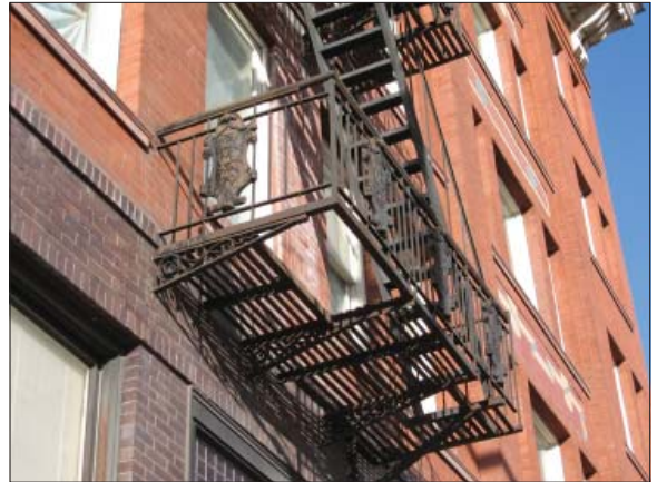
Historic fire escapes, such as the one at 379 S. Main Street, can be decorative as well as functional.
