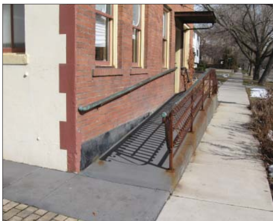
This accessibility ramp is successfully integrated with the historic building both in scale and materials.
