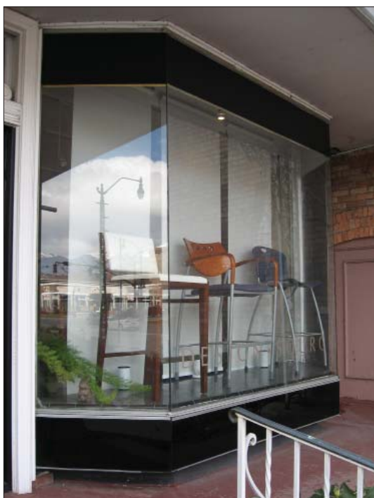
The Carrara glass is a distinctive characteristic of the storefront at 432-434 E. South Temple Street.
